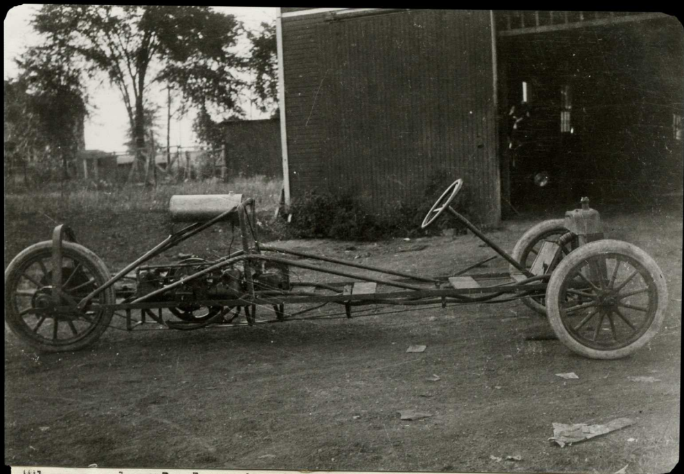
Three wheeled auto built by cousin Wm Edwards from spare parts of farm machinery. (1902-3)
